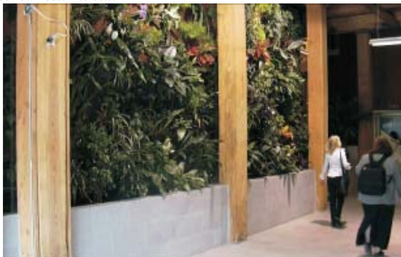
This biowall is 8 m wide by 3.6 m high for a total surface area of 28.8 sq.m. (only a portion of the wall is shown above). The system filters the air in the lobby. The cleaned air then diffuses through the rest of the JAS Robertson Building in Ontario, Canada.
